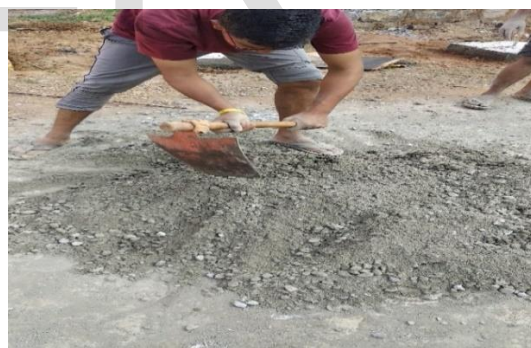
Figure 5. Dry mixing of materials
