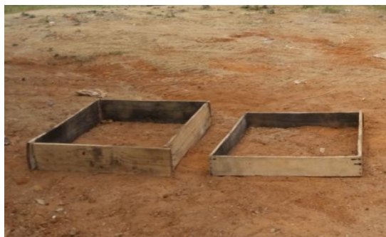
Figure 3. Moulds for Casting
