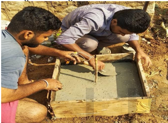
Figure 7. compaction and finishing of the mix
