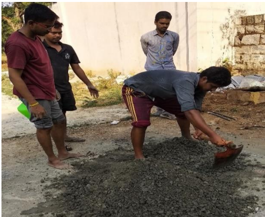
Figure 6. Mixing of constituent materials
